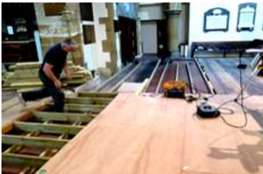
Constructing platform and installing wiring
